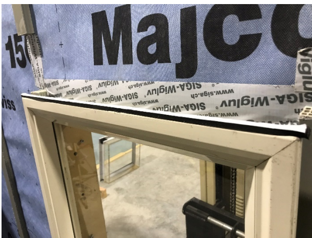
Figure 5. Application of foam tape on top of window.
