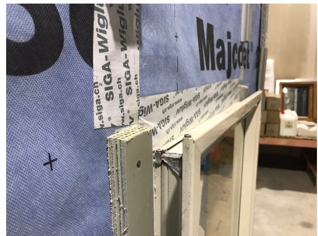
Figure 4. Sample window taped to underlay system.
